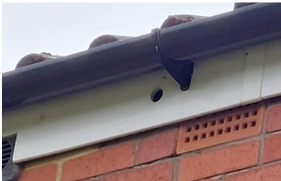
Plate 4.5: Gap in barge board on southern elevation
