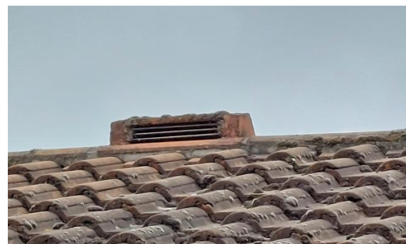
Plate 4.8: Example of vent on ridge tile
