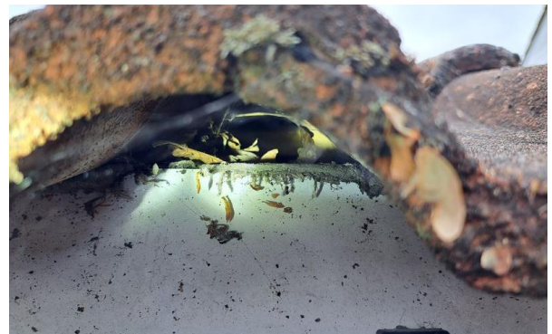
Plate 4.6: Gap underneath lower tile
