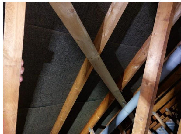
Plate 4.10: Example of felt sarking in good condition
