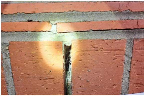
Plate 4.3: Example of weep hole
