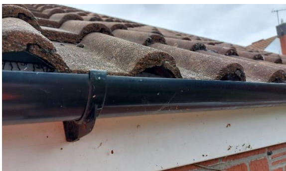
Plate 4.7: Gaps beneath lower tiles partially blocked by guttering
