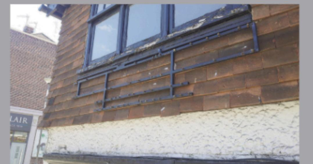
built up steel lettering, spanning 1400mm
