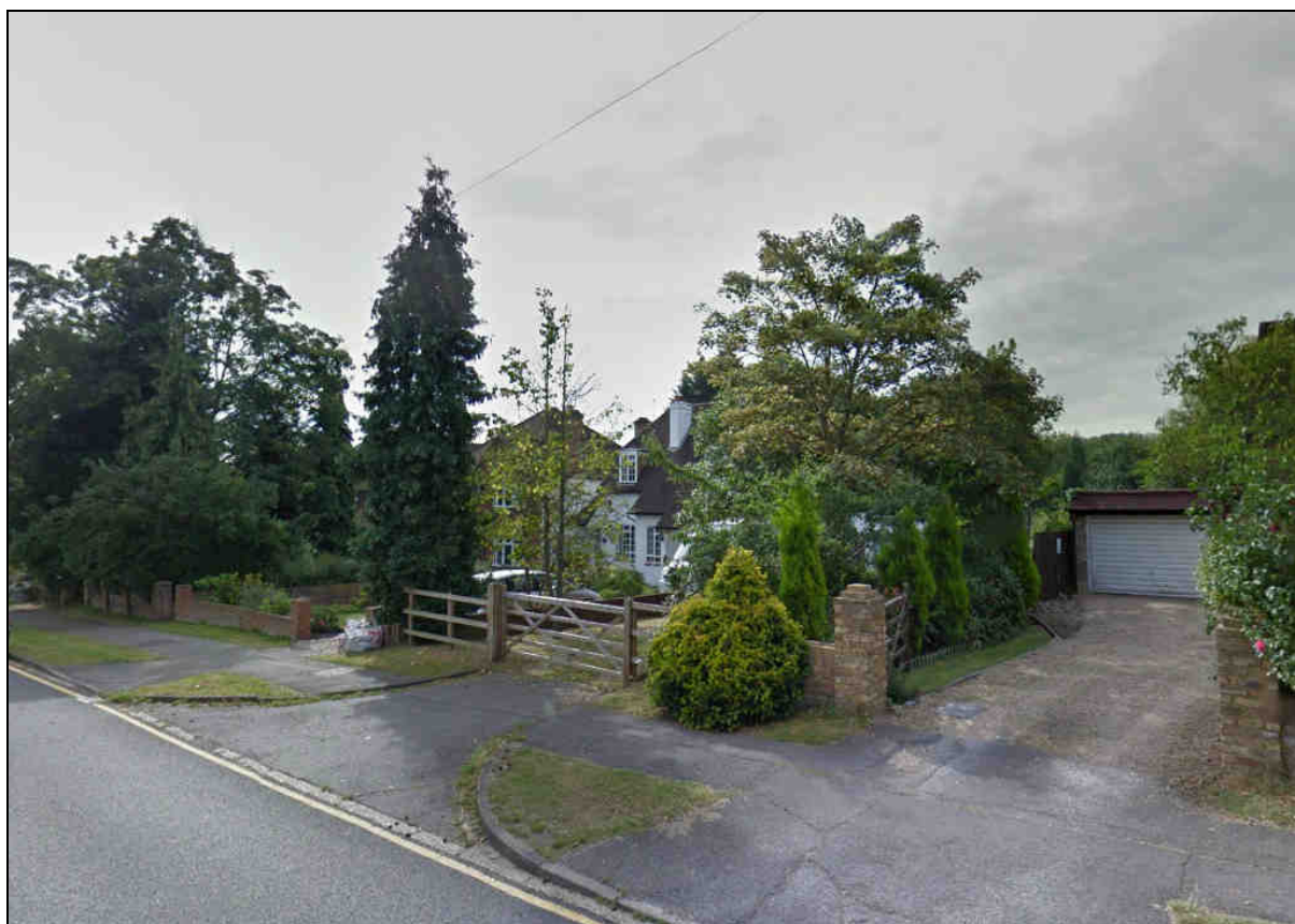
Photograph 5 – No 22 views from in front of No 20 Warren Road
