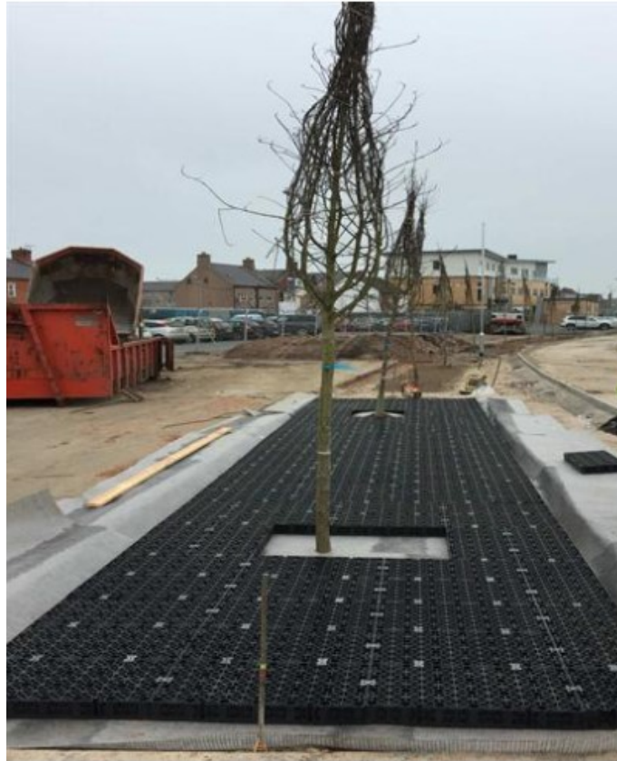
The surface of the tree pit is first covered by the ArborRaft cellular grid
