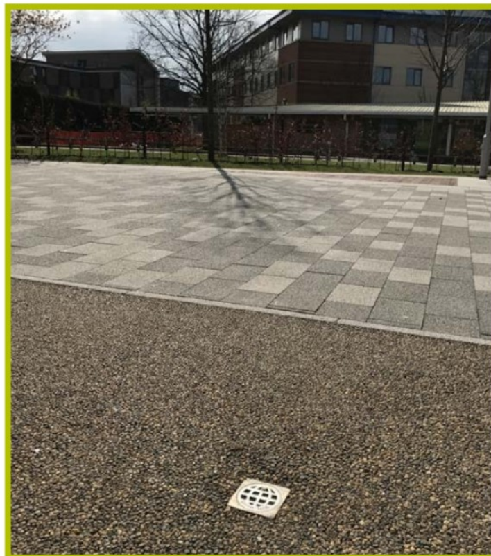
The final finish can be created with a variety of surfaces provided they are porous
