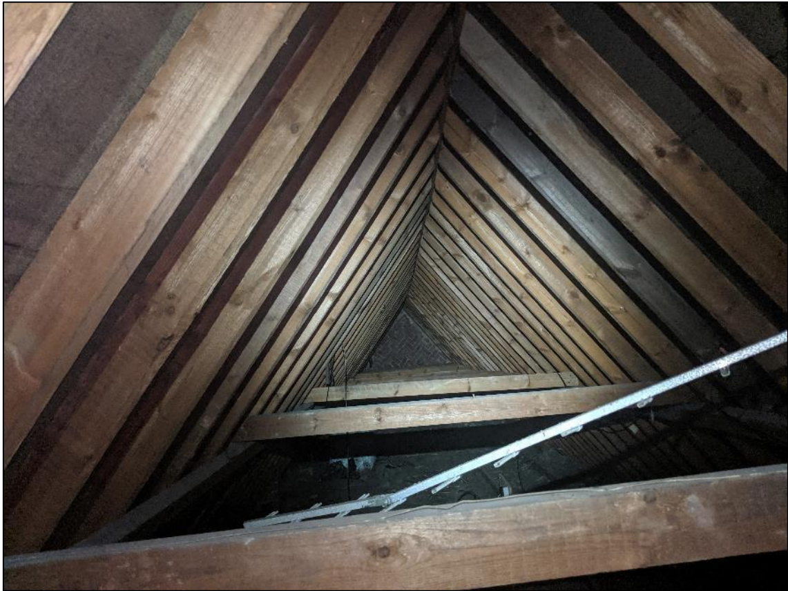
Photograph 2: Showing interior of the main void.
