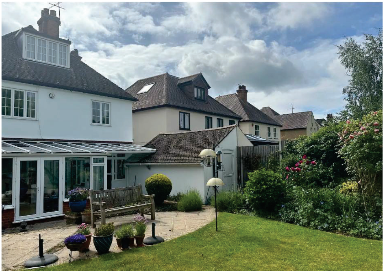
Figure 5: View of Application site from the garden of No.17 Kewferry Road
