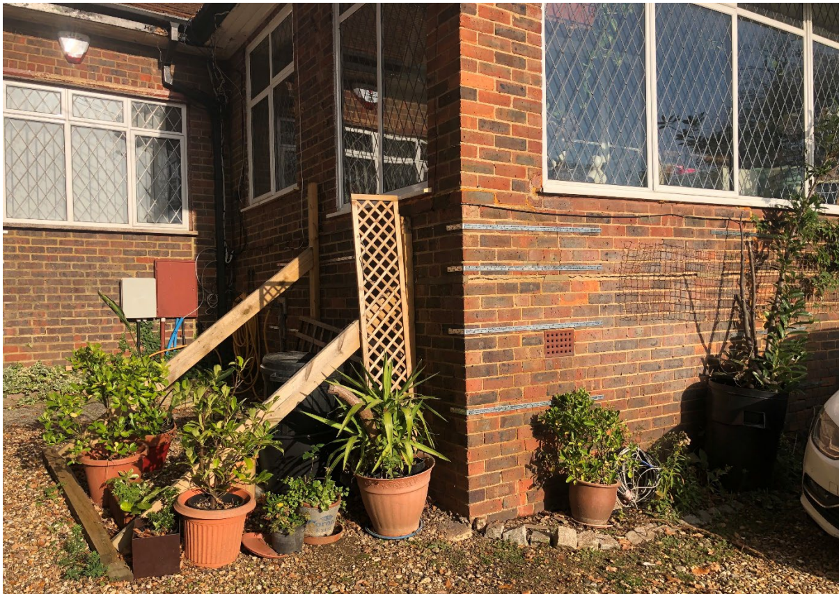
Strapping and propping to existing house
