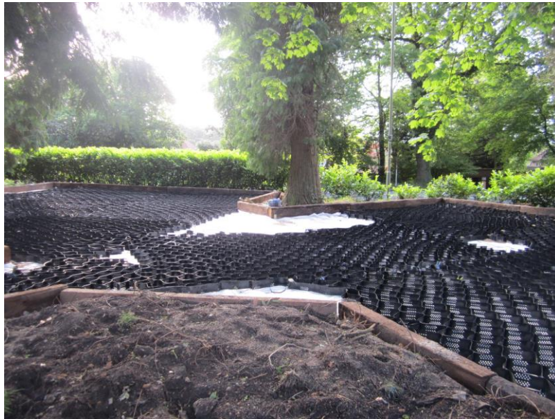
Image 14: A geo-textile membrane is laid across the sand bed and the cellular confinement system stretched and pinned across the surface area before being filled with no-fines aggregates.
