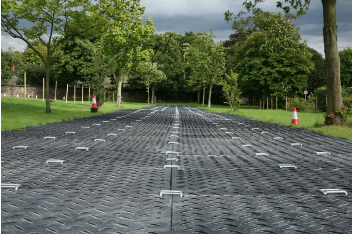
Image 17 - Ground protection, interlocking mats image: Photo shows the use of heavy duty interlinking plastic ground protection for temporary ground protection close to trees
