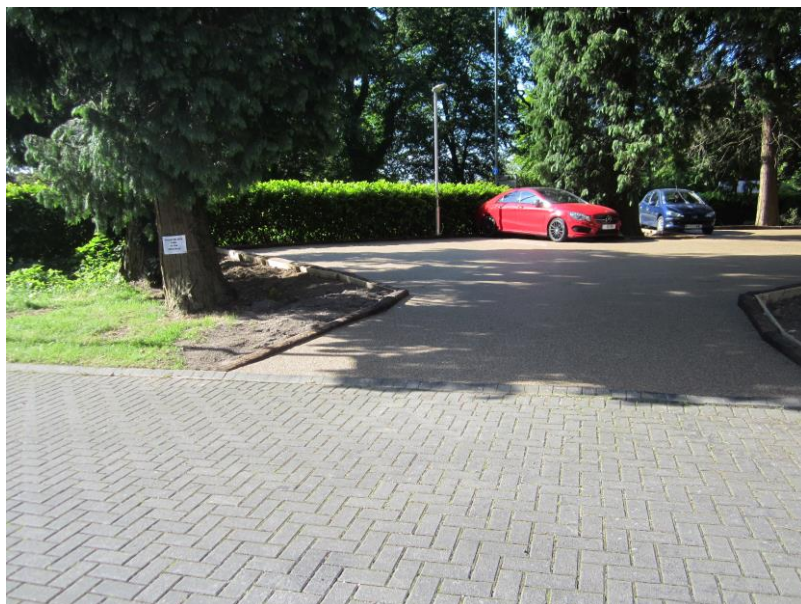
Image 15: The finished porous surfacing is then laid and the edges pinned to create an above-ground parking system.
