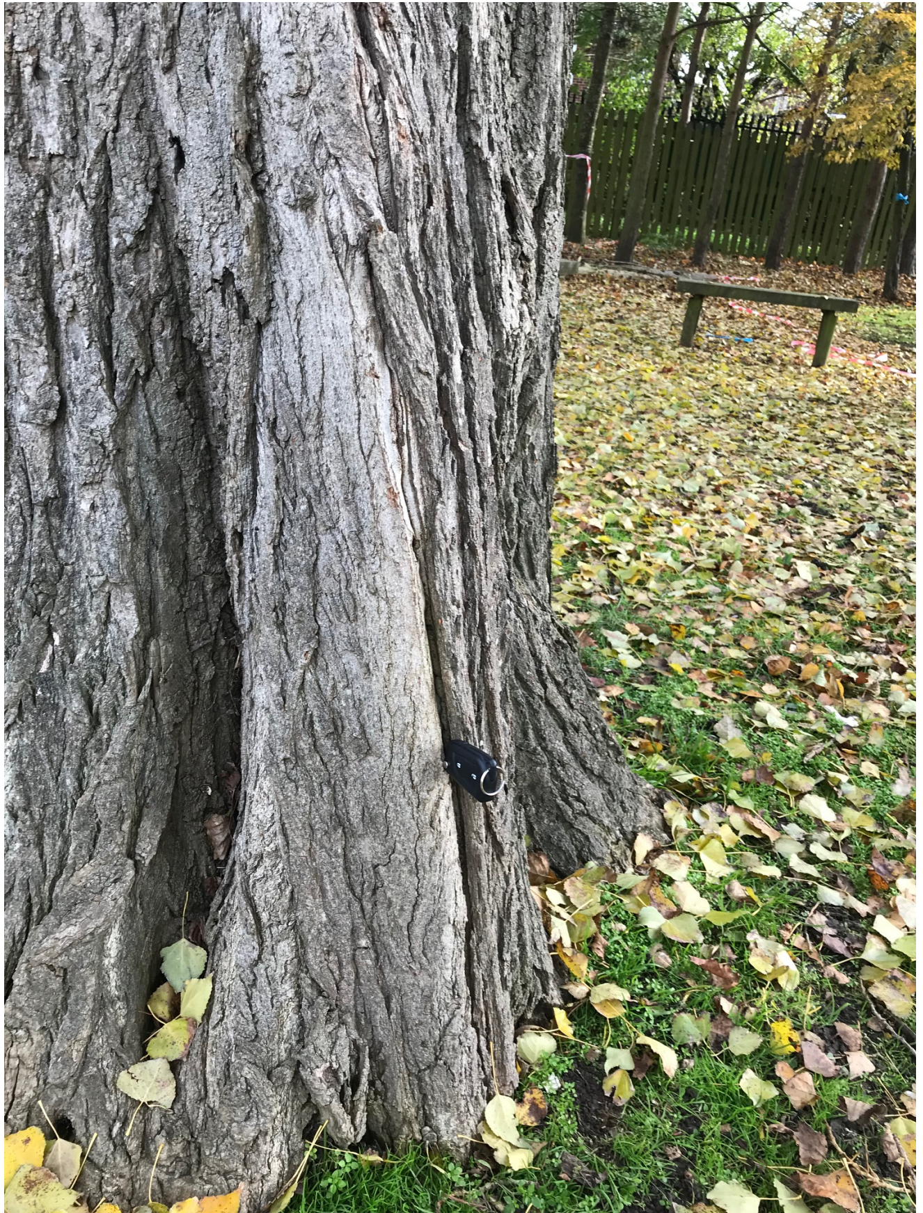
Photo 10: Tree 6: Vertical crack to western flank.
