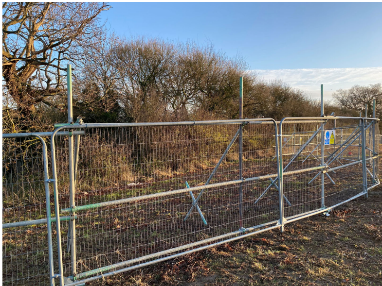
Photograph 1: showing example of TPF erected to the correct specification
