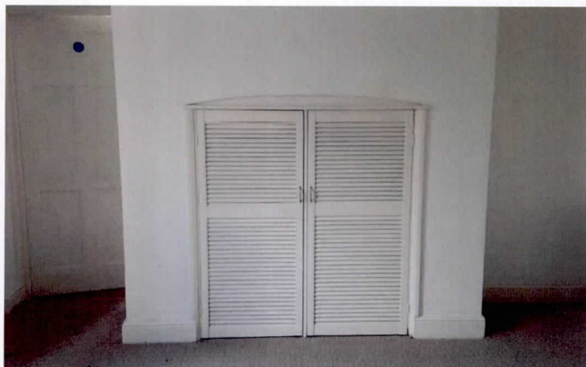
Appendix 5.12: Removed fireplace with cupboard infill
