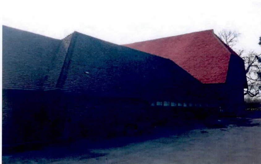
Appendix 5.31: North elevation of 3 Manor Court with the Great Barn behind
