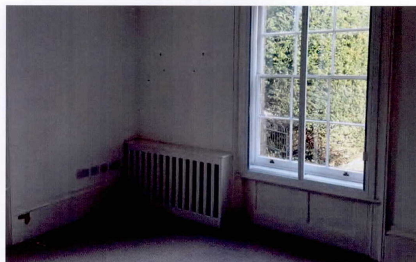
Appendix 5.14: Remaining historic fabric of under window panel and reveal
