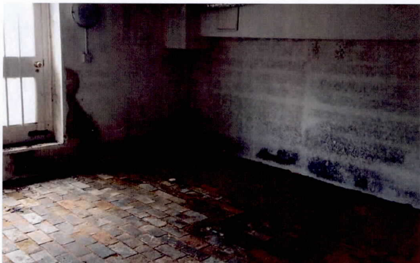
Appendix 5.15: Surviving room and floor within basement
