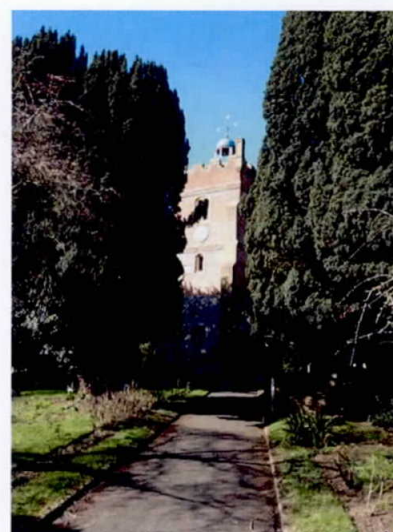
Appendix 5.35: Grade II* Church of St Mary
