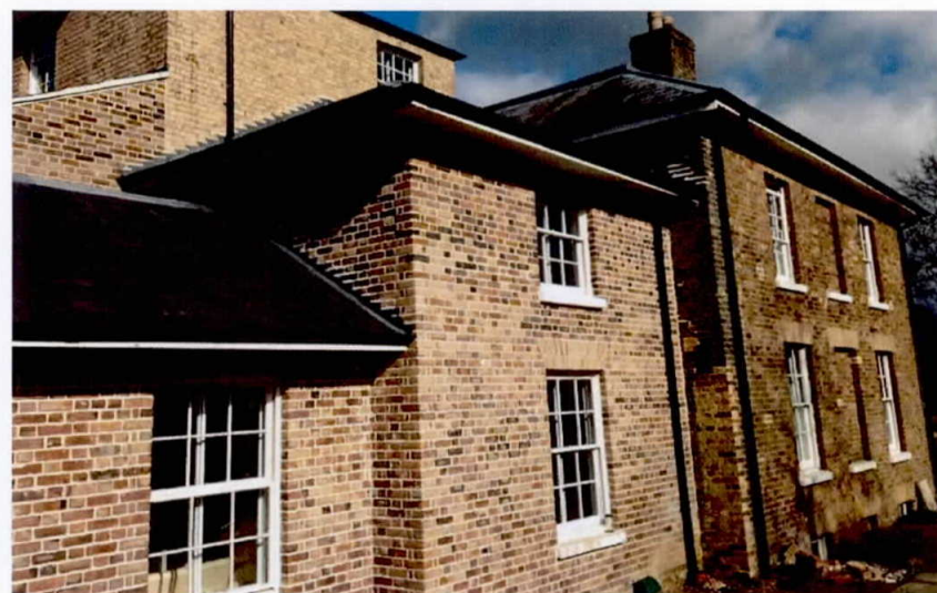
Appendix 5.4: South elevation, showing 1980s extensions, to Manor Court
