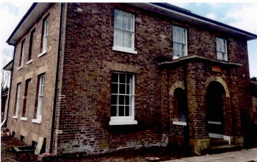
Appendix 5.2: Front (east) elevation of Manor Court
