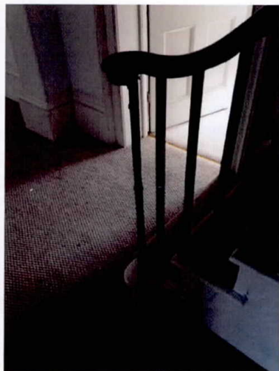
Appendix 5.10: Ground floor staircase
