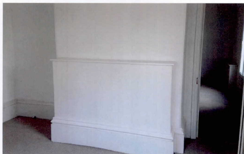
Appendix 5.9: Typical boxed in fireplace at Manor Court
