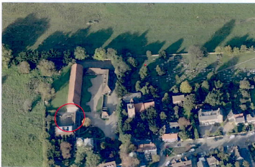
Fig 5: Map showing aerial view of the application building, Manor Lodge
