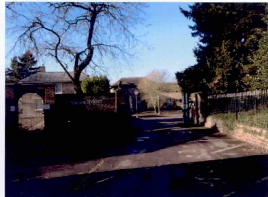
Fig 8 The entrance to Manor Court
