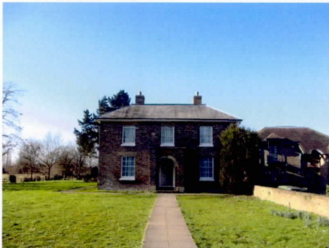
Fig 1: View of Manor Lodge from the eastern side
