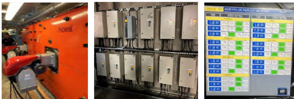
Figure 33. Existing Boilers, CHP, VSDs and VSD time schedules
