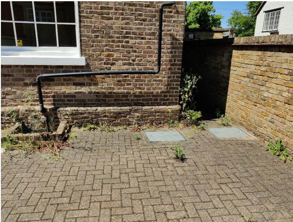
Below ground drainage manholes to rear.
