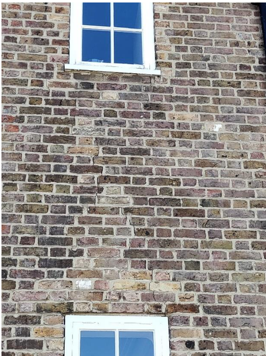
Left side ground and first floor window
