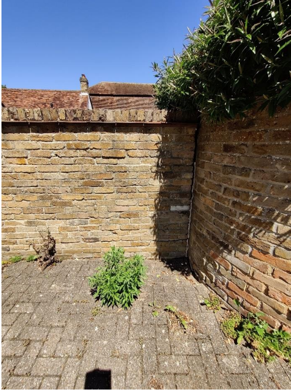
Left side boundary wall at junction with curved rear wall.
