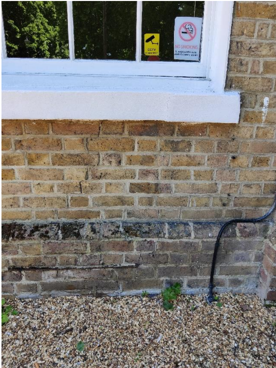
Front ground floor window cill
