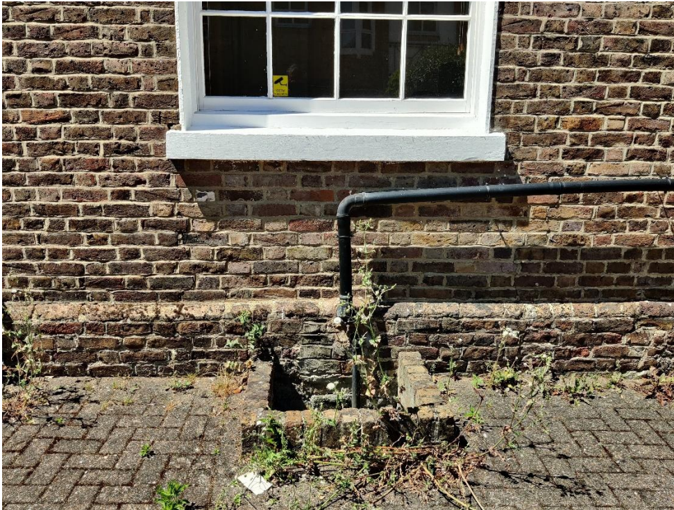
Rear right ground floor window cill.
