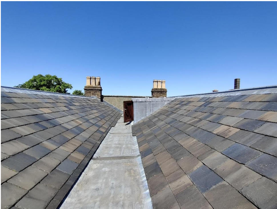
Internal valley gutter to roof.
