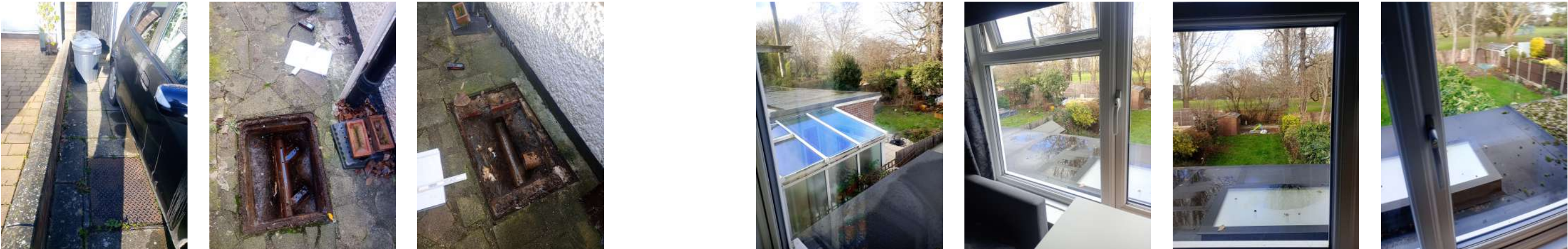
Manholes on site.
