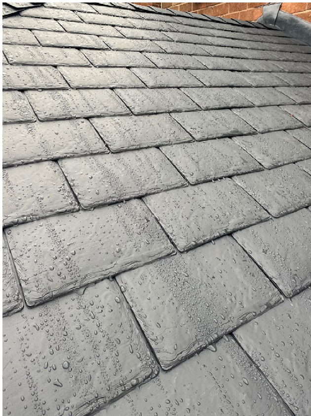
SUPASLATE ECO LINE PLASTIC ROOF TILE
