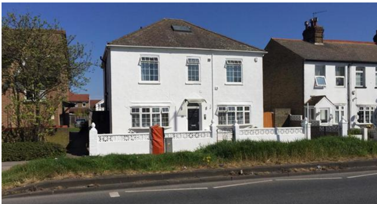
Image 4: 46 Bath Road (frontage (taken April 2020))
