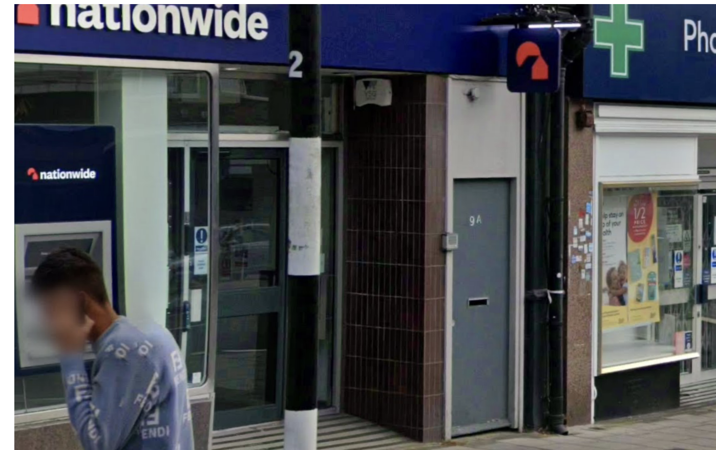
IMAGE OF ENTRANCE DOOR RECESS WHERE DUAL CABINET WILL BE FITTED TO RIGHT HAND SIDE
