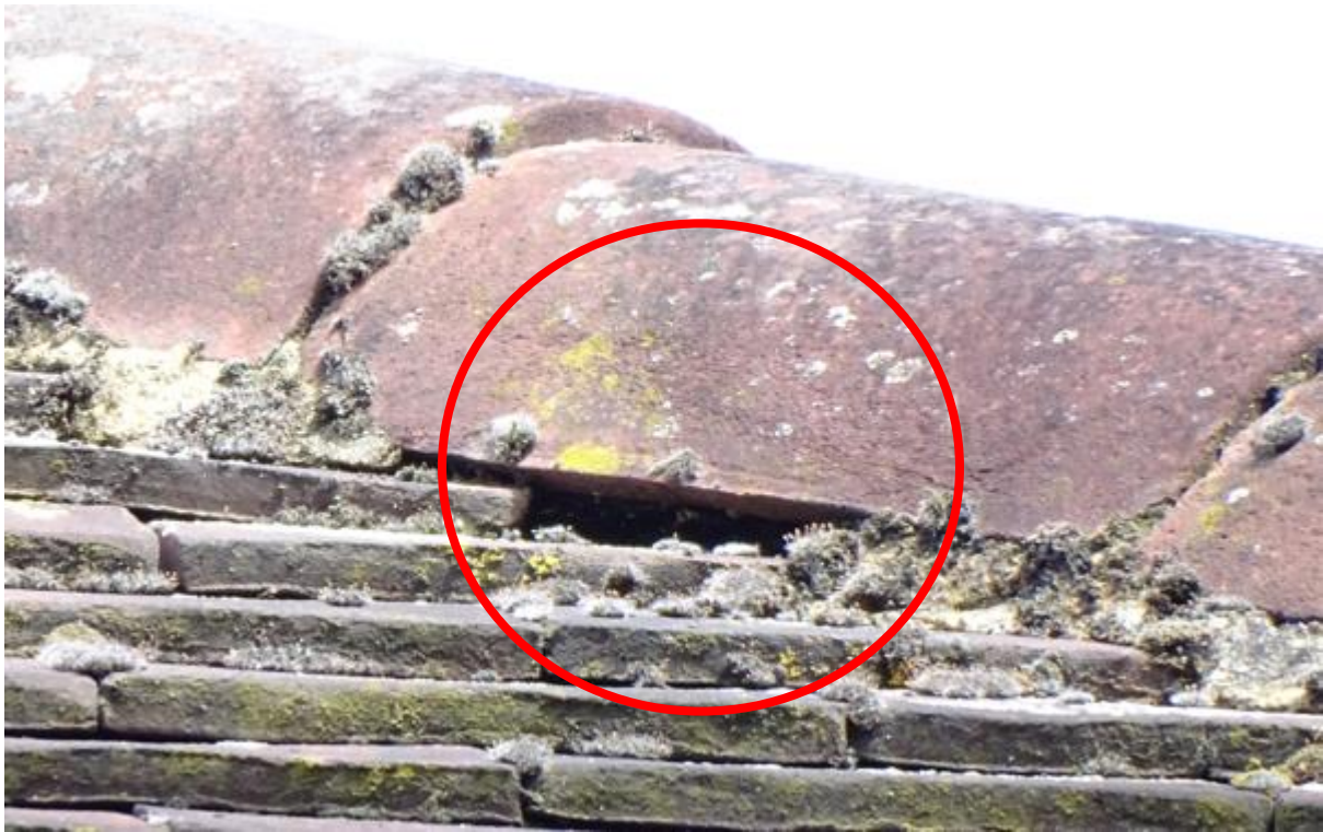
Image 3 – Gap within the North facing elevation hop coverings which looks to offer likely shelter opportunities for crevice dwelling bats
