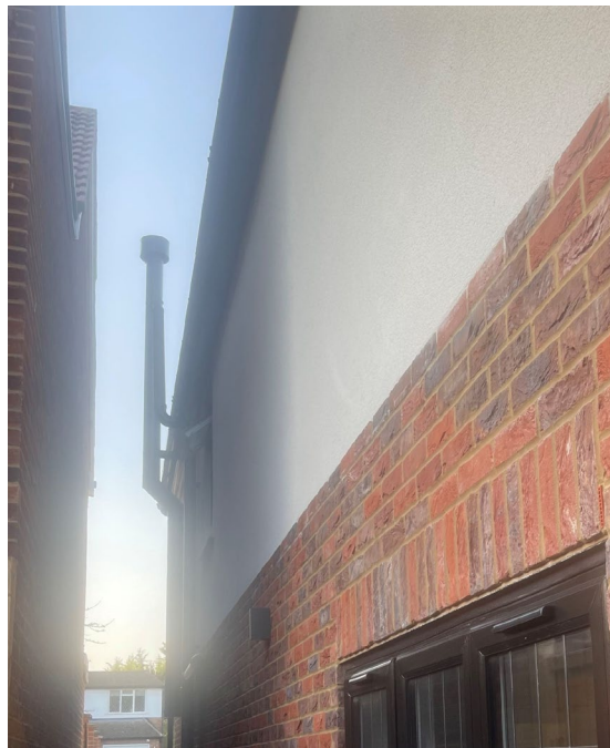
Figure 3 - Wall flue as built
