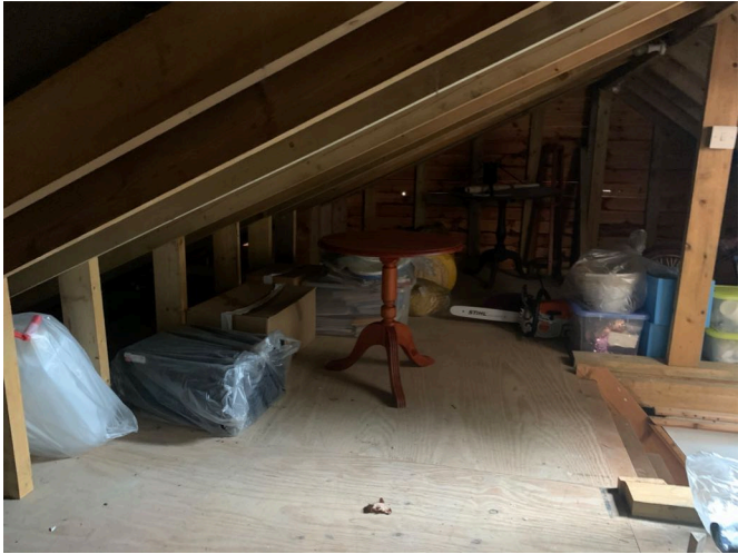
Interior views of the existing outbuilding attic
