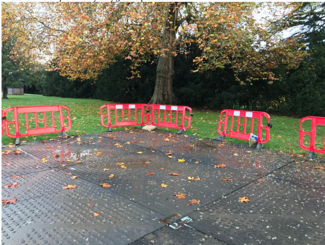
Photo 2. An example of heavy-duty ground protection.
