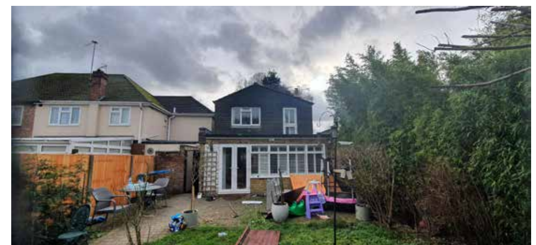
Rear elevation of existing house
