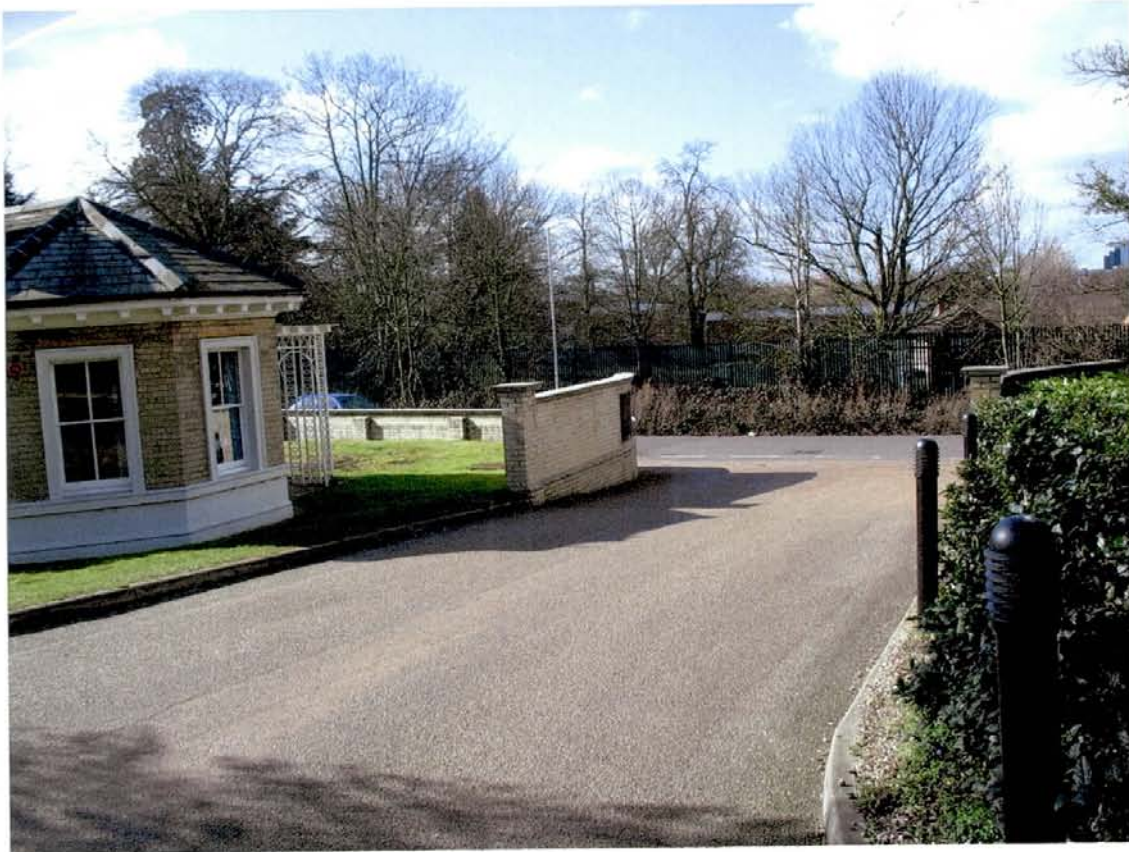
Fig 2: View from the access looking west towards Vine Lane showing southern wall to be lowered to plinth level
