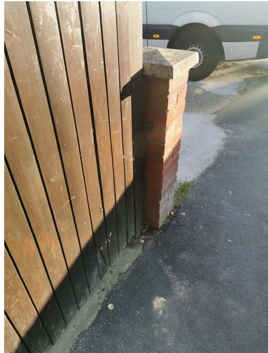
P2 -Existing wall at NW site boundary - towards the adjacent property at 160 Ashford Avenue - 40mm distance between existing wall and site boundary
