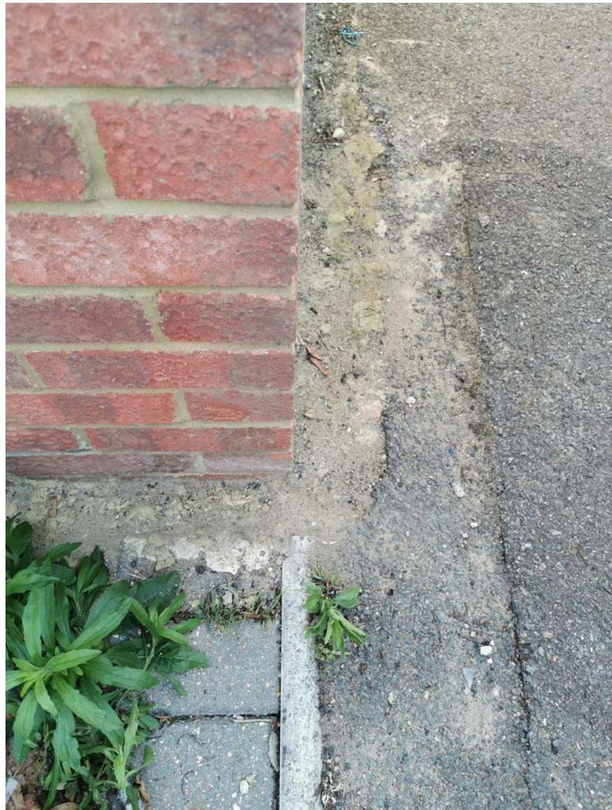
P1 - Existing wall at NE site boundary - 40mm distance between existing wall and site boundary
