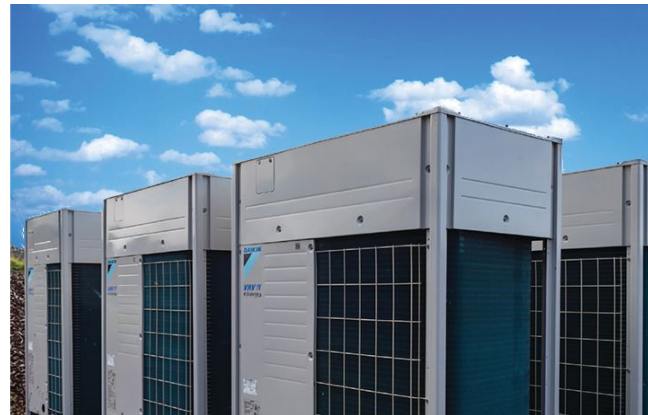
Figure 10: (Top) ©Mitsubishi, Y Series VRF Standard Heat Pump (YNW) (Bottom) ©Daikin, example VRF system on roof
