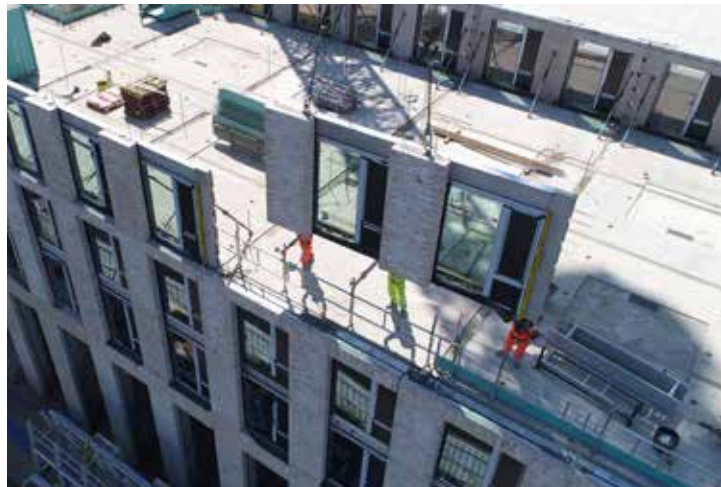
Example off-site facade construction
