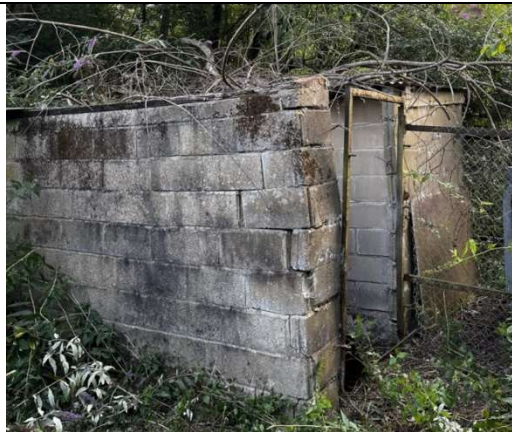
Gaps in masonry
