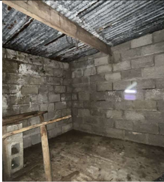
Gaps between roof and brickwork
