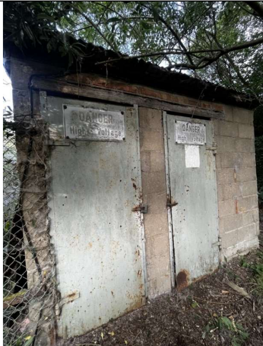
Gaps above doors – audible hum of equipment.
