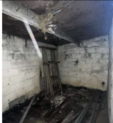
Plywood roof in poor condition with splits and holes
