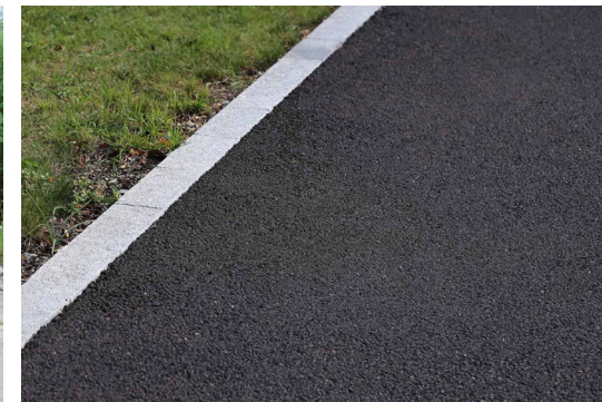
Black Top Tarmac with PCC roadkerb for pedestrian access footway
