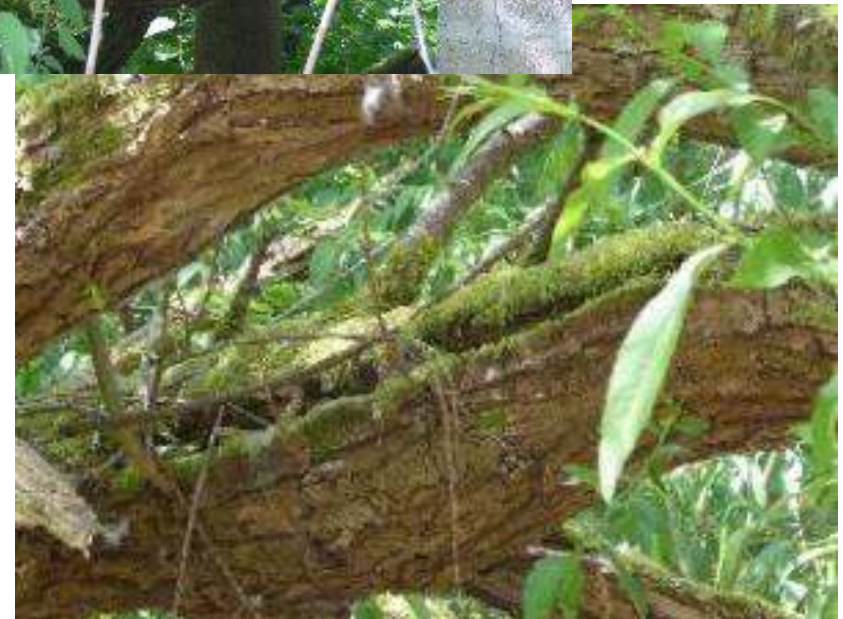
T17 Multiple stem cracks including hazard beams between 0.5 and 2m, east facing. Moderate potential.
