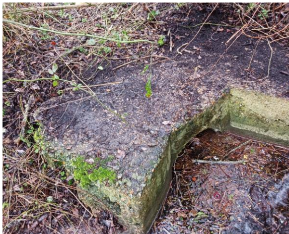
(a) Pipe inlet
