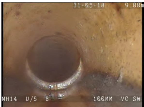
B_MH14X_f80fcc4a-b6ef-4fc9-a41e-e90103d837d1_20180604_145211_035.jpg, 00:01:13, 10.00m Joint displaced, medium
