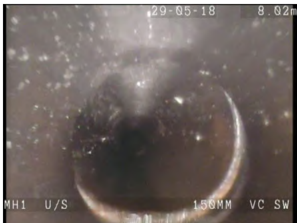
MH3X_a3ddf67a-6157-40fe-801c-e0e08bedef87_20180604_105126_505.jpg, 00:00:36, 8.10m Joint displaced, medium
