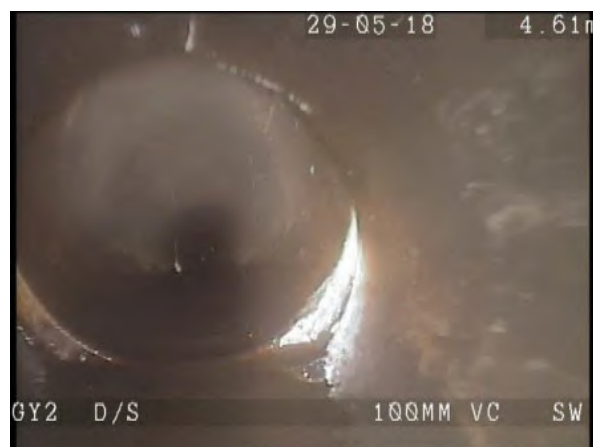
GY2X_a79ea17b-9a1f-4af5-83d4-555353067472_20180604_114230_449.jpg, 00:00:34, 4.70m Joint displaced, medium
