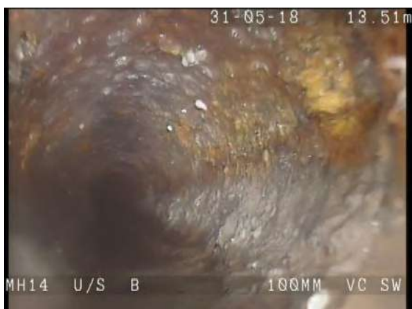
B_MH14X_18d6d96b-3466-4bf2-97b0-6d6743690ace_20180604_150518_290.jpg, 00:01:44, 13.50m Material changes to cast iron
