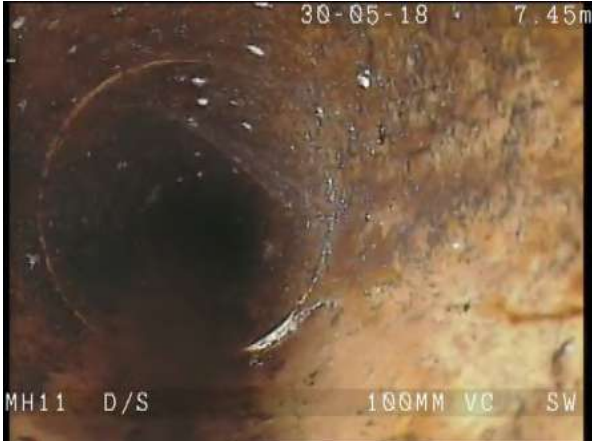
MH11X_45b8ff6e-664e-4988-89f3-78e69c1534ea_20180604_1 30155_767.jpg, 00:00:57, 7.50m Fracture, longitudinal at joint at 4 o'clock
