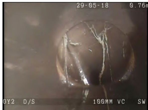
GY2X_33c5c1ea-f169-4d8f-ada0-a495ecdef433_20180604_114148_482.jpg, 00:00:12, 0.80m Joint displaced, medium
