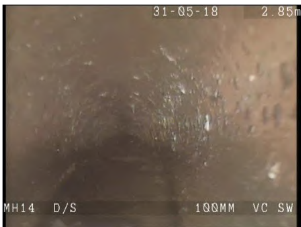
MH14X_cb3f99e3-0051-486d-941d-521f01aa8701_20180604_154912_875.jpg, 00:00:22, 2.90m Water level, 20% of the vertical dimension
