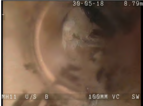
B_MH11X_ece2156b-2a64-47e8-81b9-f28b627ce6dd_20180604_131600_646.jpg, 00:01:07, 8.80m Settled deposits, coarse, 50% cross-sectional area loss
