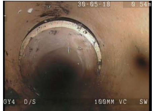
GY4X_fb7ebc75-bacb-4bc7-9aa2-9c46b27d4ab2_20180604_132856_232.jpg, 00:00:18, 0.60m Joint displaced, medium
