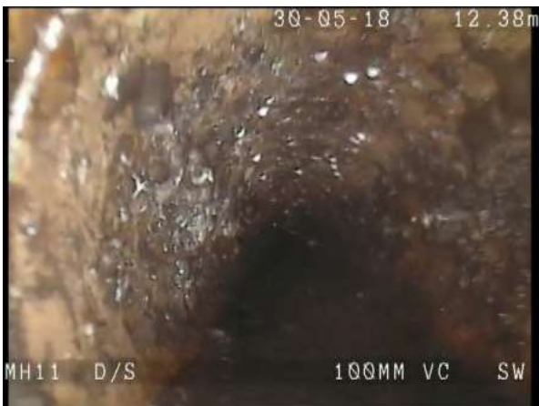
MH11X_c36e24ac-677f-42e1-8109-ac41a0b01cfb_20180604_1 30344_193.jpg, 00:01:23, 12.40m Settled deposits, fine, 5% cross-sectional area loss, start
