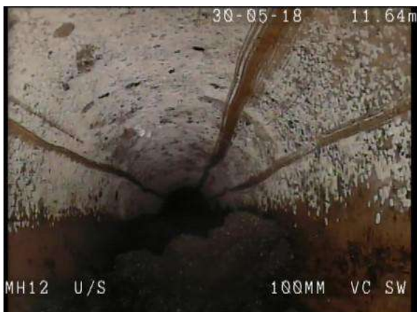
U_S MH12X_2bbc4dde-a064-4af7-8145-a1a1beeace39_20180604_ 133947_373.jpg, 00:01:21, 11.70m Settled deposits, fine, 10% cross-sectional area loss
