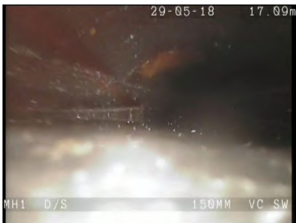
MH1X_df6d95d8-c6d1-46e8-9f07-eb4d7e02ebd3_20180604_1 10121_139.jpg, 00:01:07, 17.10m Water level, 30% of the vertical dimension
