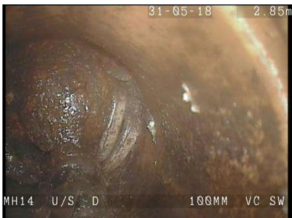
D_MH14X_a3025a4a-48bc-453f-b890-f5ff270501e4_20180604_154048_176.jpg, 00:00:45, 2.90m Other obstacles from 4 o'clock to 8 o'clock, 40% cross-sectional area loss
