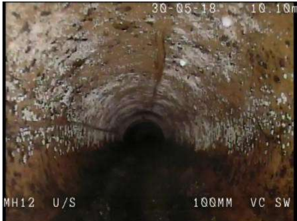
U_S MH12X_427be56e-b667-4e80-a128-1737d92584ef_20180604_ 133524_873.jpg, 00:01:11, 10.10m Settled deposits, fine, 5% cross-sectional area loss, start
