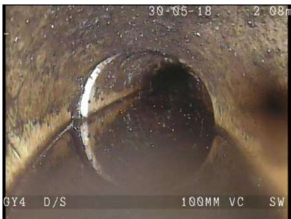
GY4X_f2a9412c-e04b-47e4-a18a-4c80e63c3138_20180604_132918_034.jpg, 00:00:28, 2.10m Water level, 20% of the vertical dimension
