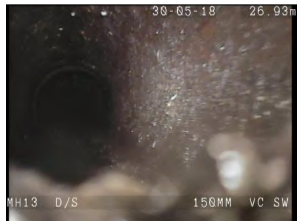
MH13X_1bfd6dfd-bb9d-4c16-adf4-dd01b0b5bb0a_20180604_140445_777.jpg, 00:02:42, 27.00m Settled deposits, fine, 5% cross-sectional area loss, start
