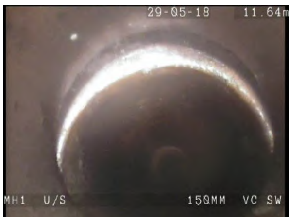
MH3X_d36944c7-39db-467e-8472-70c44a59c664_20180604_105151_525.jpg, 00:00:48, 11.60m Joint displaced, medium
