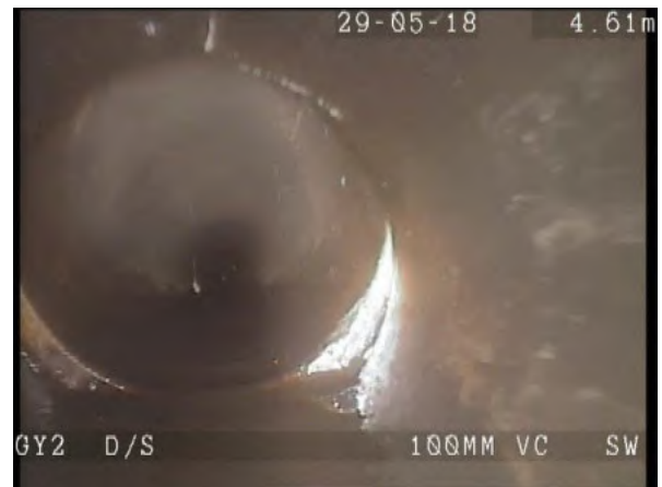
GY2X_a79ea17b-9a1f-4af5-83d4-555353067472_20180604_114230_449.jpg, 00:00:34, 4.70m Joint displaced, medium
