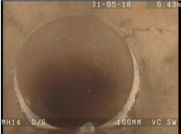
MH14X_168c0c70-77c0-4d60-9b76-dbb6a92cb306_20180604_154812_244.jpg, 00:00:09, 0.50m Crack, longitudinal at joint at 2 o'clock
