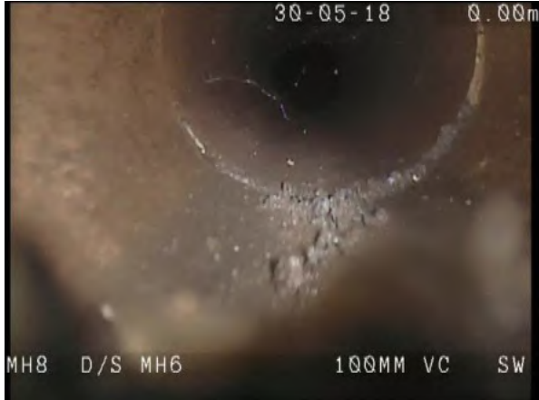
MH8X_bee0a5bd-6969-44a3-b524-0a7d76b6459c_20180604_1 20848_871.jpg, 00:00:06, 0.10m Settled deposits, fine, 5% cross-sectional area loss
