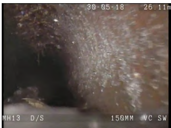
MH13X_5646dd2b-e2fd-4983-bc3b-baadbd282d9a_20180604_140400_848.jpg, 00:02:36, 26.10m Settled deposits, coarse, 10% cross-sectional area loss
