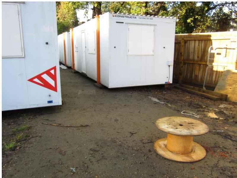
Image 6 - Containers and welfare units within RPA 2: Storage containers and welfare units may be placed and supported on above-ground structures such as pads, blocks and scaffolding.
