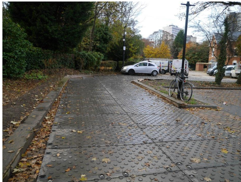
Image 5 - Ground protection mats over hard surfacing: Interlocking ground protection mats can be used to reinforce hard surfacing to support the anticipated load of plant machinery
