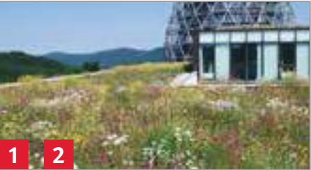
Extensive and intensive green roof
