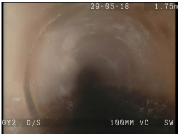
GY2X_d3e3e17c-9730-48b7-b2a5-2de544580fdd_20180604_114259_842.jpg, 00:00:19, 1.80m Crack, circumferential from 12 o'clock to 12 o'clock
