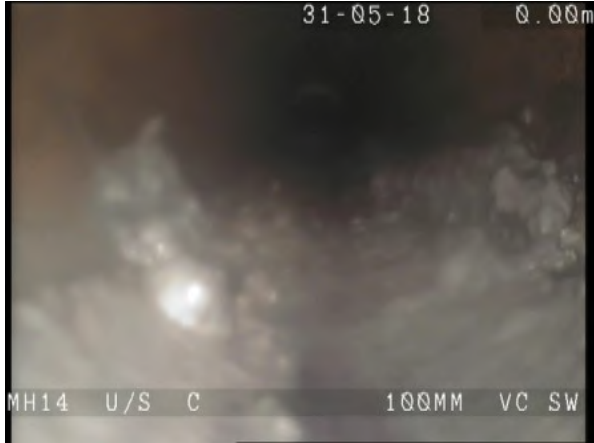
C_MH14X_680d6f3c-0fea-4b52-9ccd-474b44ce4e91_20180604_151707_649.jpg, 00:00:07, 0.10m Settled deposits, fine, 5% cross-sectional area loss
