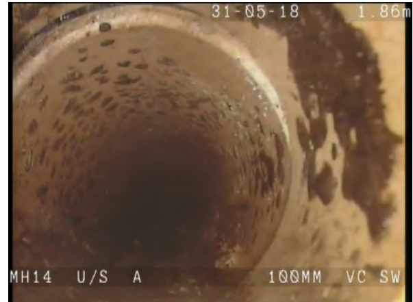
A_MH14X_0ebe5ef9-0fe6-42d8-a01f-5de9df510e83_20180604_143440_621.jpg, 00:00:16, 1.90m Joint displaced, medium
