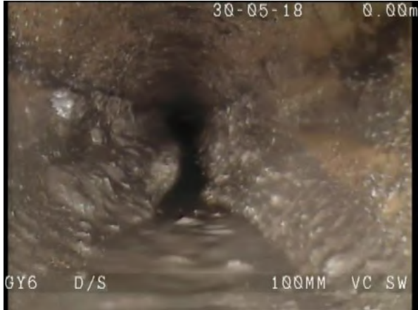
GY6X_4f11b5a9-0457-4edd-8c58-6809d6ef90ec_20180604_141001_233.jpg, 00:00:05, 0.10m Settled deposits, fine, 20% cross-sectional area loss, start
