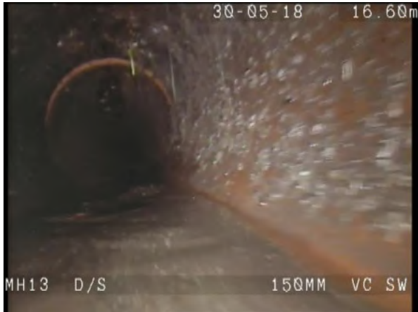
MH13X_3a5ea860-e9c1-4aa8-bd1c-61770eea8ec1_20180604_140213_355.jpg, 00:01:44, 16.60m Settled deposits, fine, 5% cross-sectional area loss, start
