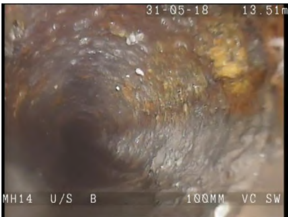
B_MH14X_18d6d96b-3466-4bf2-97b0-6d6743690ace_20180604_150518_290.jpg, 00:01:44, 13.50m Material changes to cast iron
