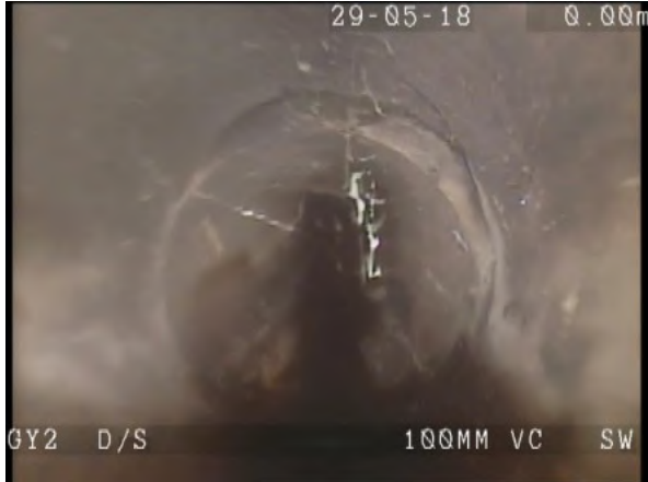
GY2X_dd061343-718e-4456-898a-1efea845b377_20180604_114119_072.jpg, 00:00:07, 0.20m Hole in drain or sewer at a joint from 11 o'clock to 3 o'clock
