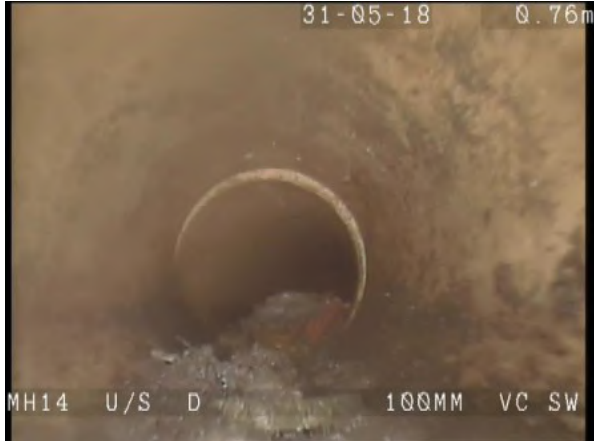
D_MH14X_b1db26ca-8089-47d0-a1ff-45bb5a26b379_20180604_152331_678.jpg, 00:00:11, 0.80m Settled deposits, fine, 10% cross-sectional area loss, start
