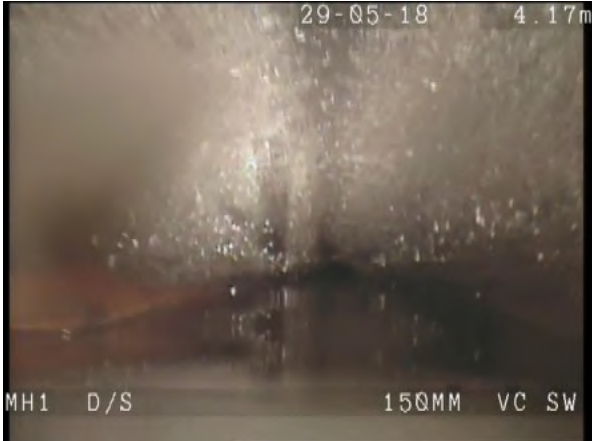
MH1X_4239433d-b5af-4ddc-a80a-48b68d4cb309_20180604_1 05613_527.jpg, 00:00:18, 4.10m Water level, 40% of the vertical dimension
