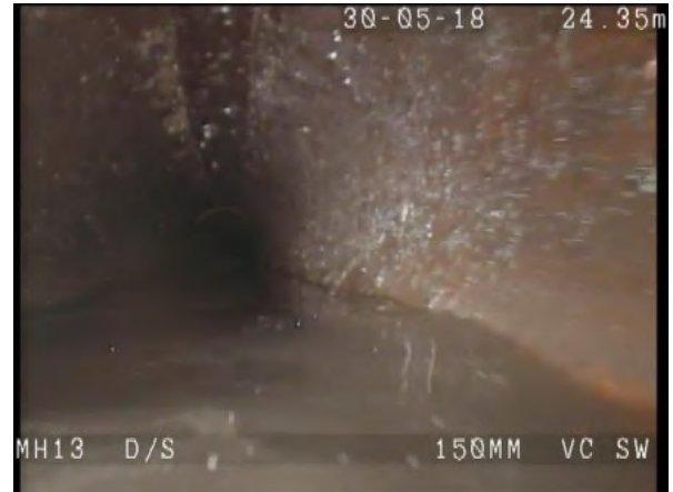
MH13X_7c3a29fa-817e-4c34-b5ab-992eafca8806_20180604_140331_807.jpg, 00:02:23, 24.30m Water level, 20% of the vertical dimension
