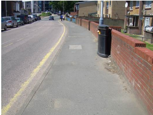
Photo 3.9 Horton Road footway (north) looking west
