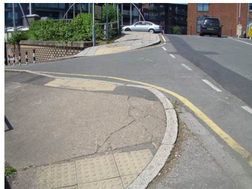
Photo 3.12 Horton Road south looking to High Street
