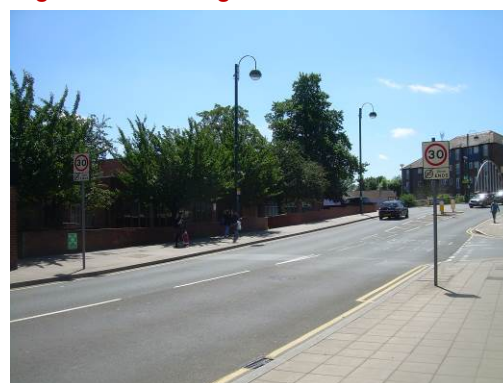
Photo 2.2 High Street looking south
