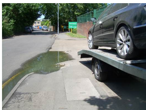
Photo 2.3 St Stephen's Road Existing ponding and obstructions
