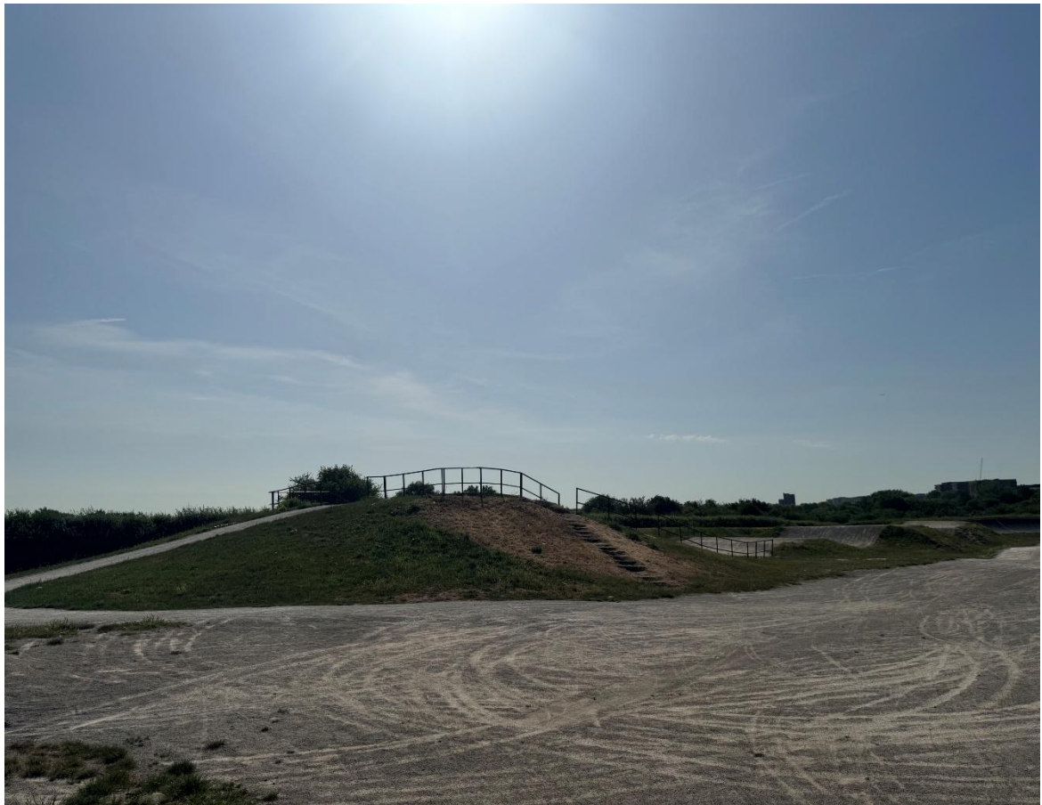
Figure 10: View of centre of the site
