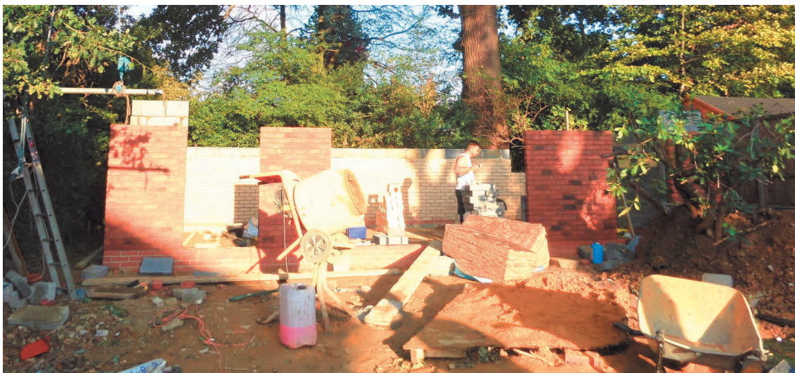
Work stopped on Friday 2 nd October 2020 after intervention of Planning Department.
