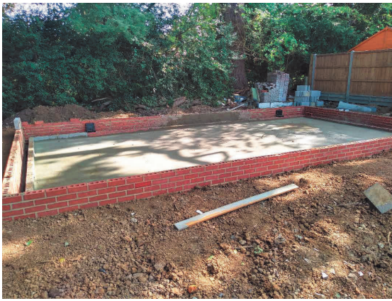
Oversite concrete poured over DPM
