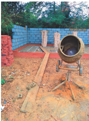
Laying of Beam & Block floor
