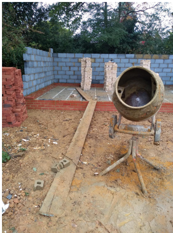
Laying of Beam & Block floor
