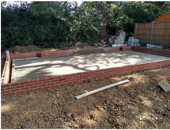
Oversite concrete poured over DPM
