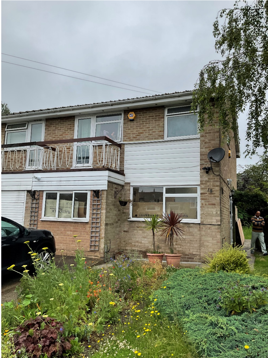
SITE PHOTOS: 18, Knoll Crescent, Northwood, HA6 1HJ
