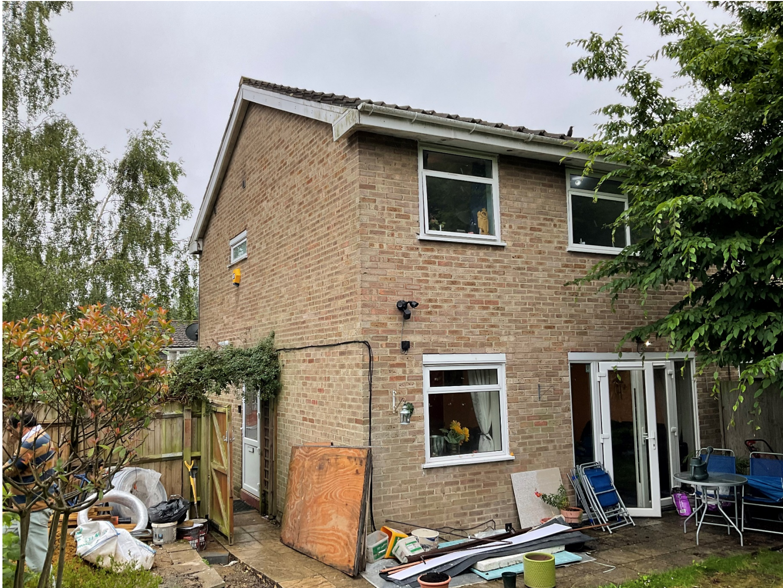
SITE PHOTOS: 18, Knoll Crescent, Northwood, HA6 1HJ
