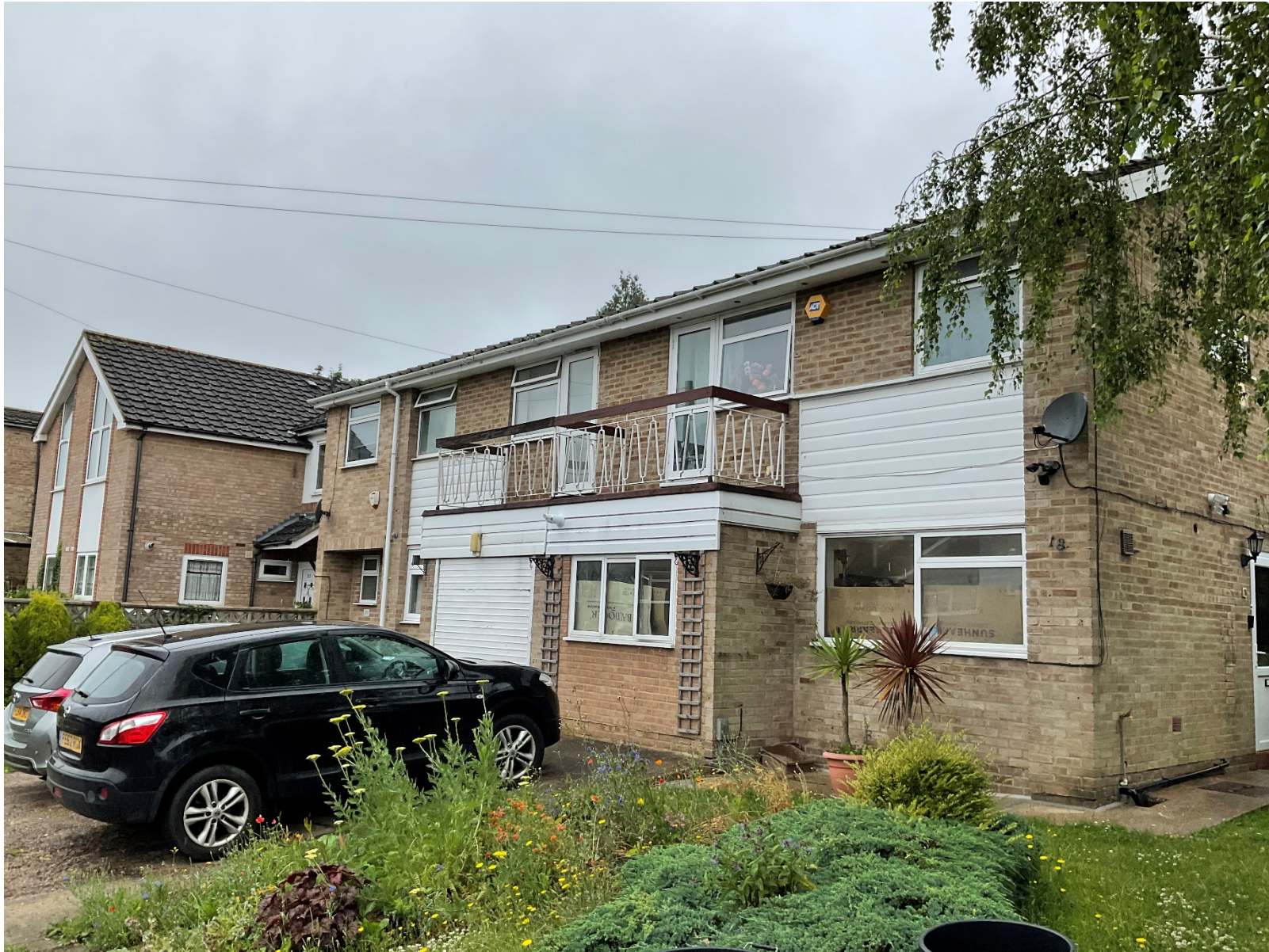
SITE PHOTOS: 18, Knoll Crescent, Northwood, HA6 1HJ
