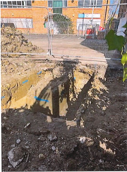
22 March 2022 - Completion of trenching with foundations of concrete laid and left to harden
