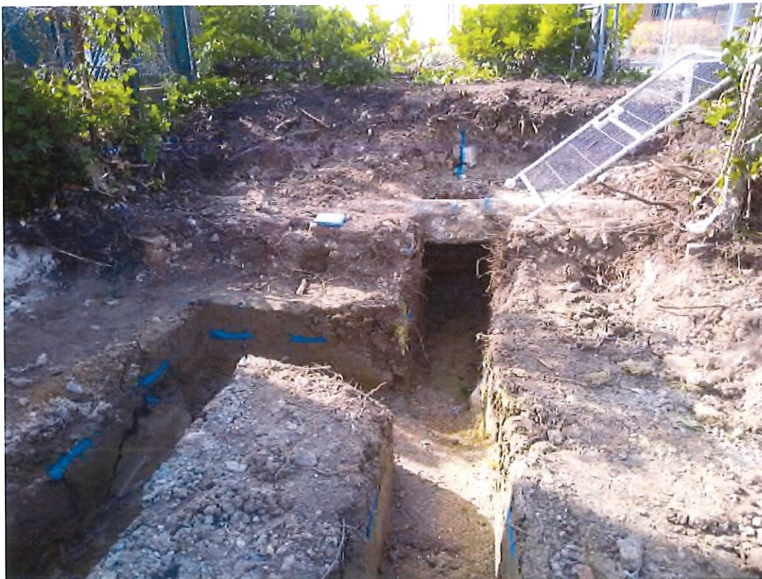
22 March 2022 - Completion of trenching with foundations of concrete laid and left to harden
