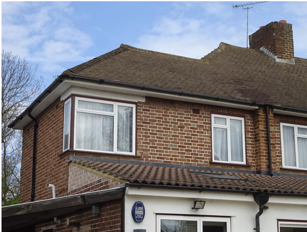
Image 1 Existing House showing matching brickwork and bonding at first floor level.
