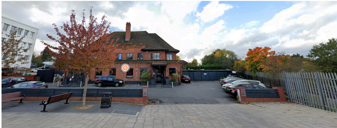
Front of existing premises showing the existing front fencing to the northern side which would be replaced
