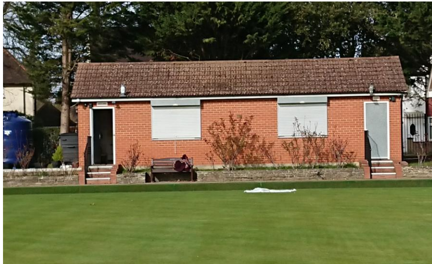
Fig 4 - Photograph of Existing Elevation
