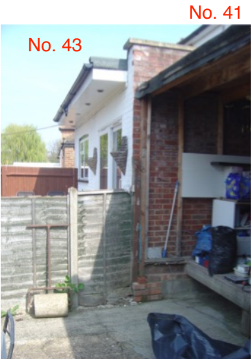
View of the neighbour's rear extension
