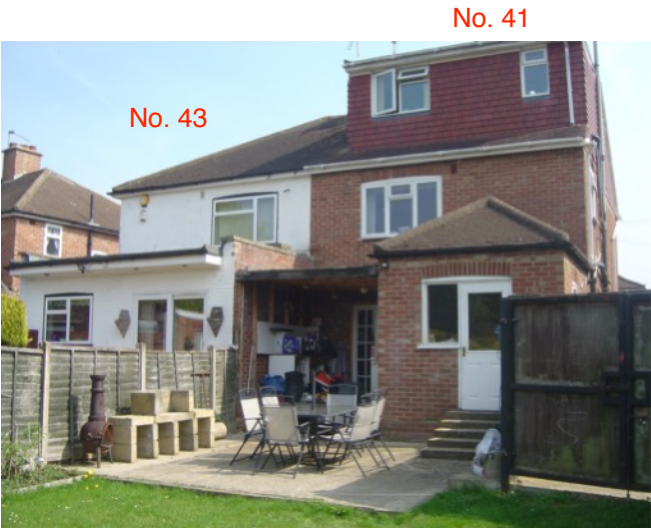
Views of the rear elevation of no. 41 from the garden
