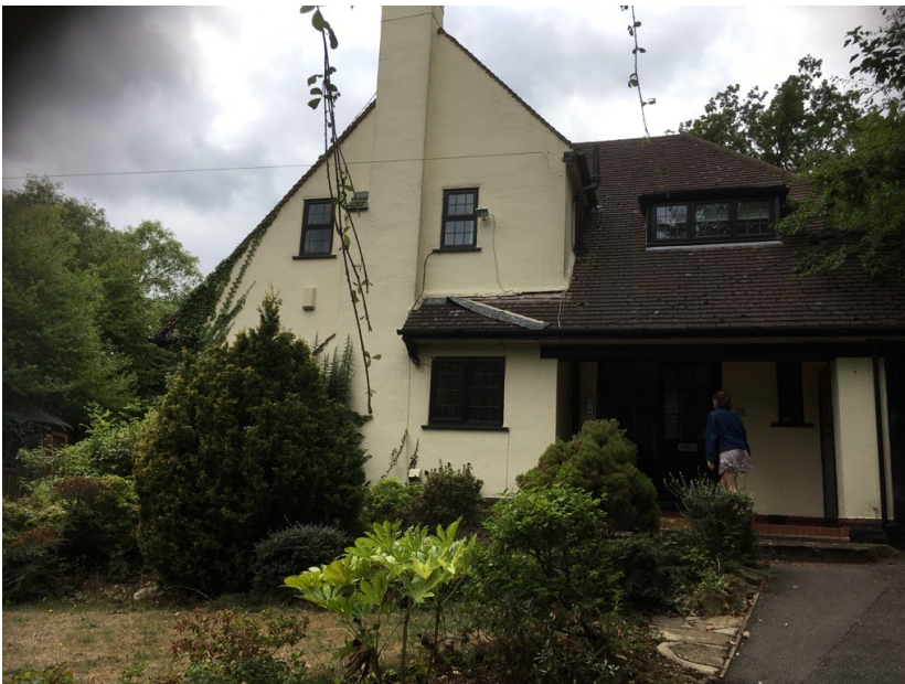
Existing East / Front Elevation onto Gatehill Rd
