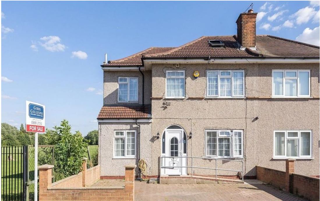
Image 1 – Front elevation of property
