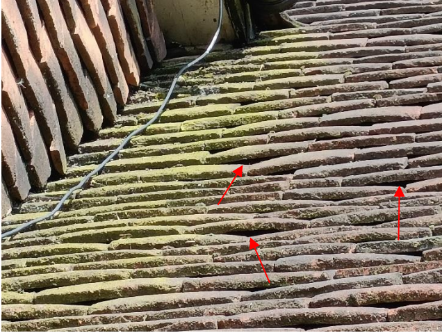
Figure 4. Example of gaps under roof tiles
