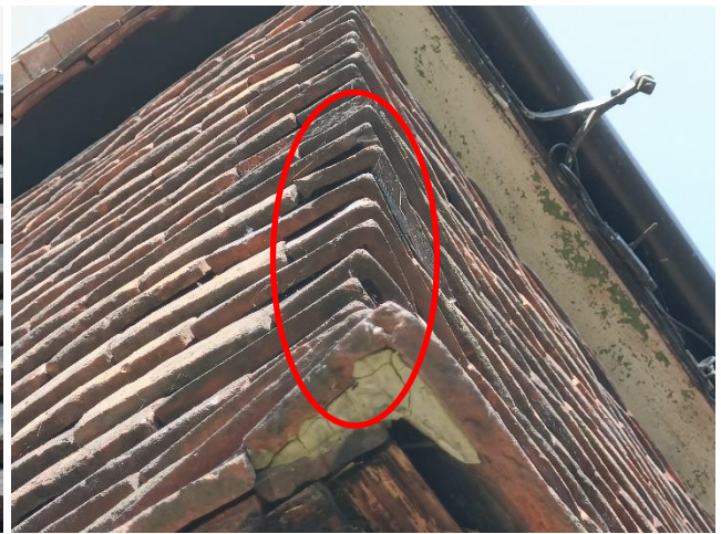
Figure 5. Example of gaps behind hanging tiles
