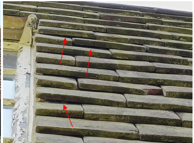
Figure 6. Example of gaps behind hanging tiles
