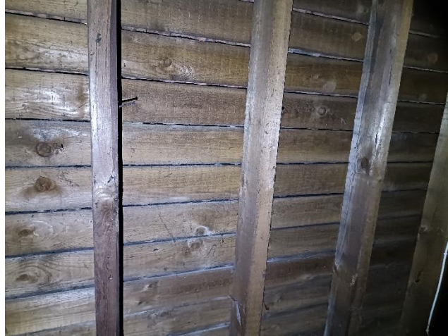
Figure 12. Example of tightly fitted weatherboarding in a good condition
