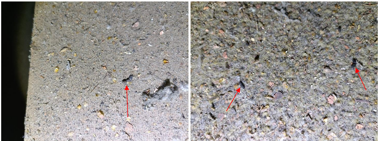
Figure 13. Example of bat droppings found during the internal inspection
