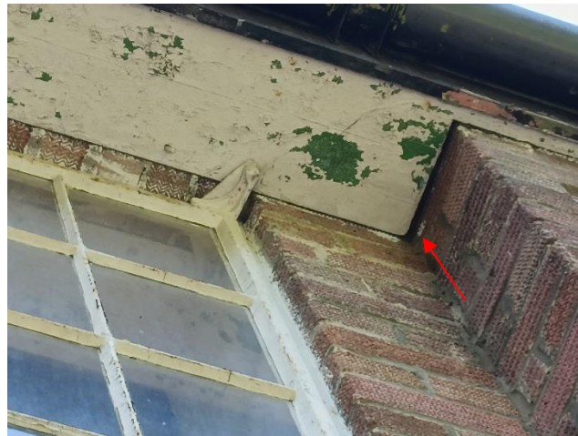
Figure 9. Example of the gaps between the soffits and the brickwork
