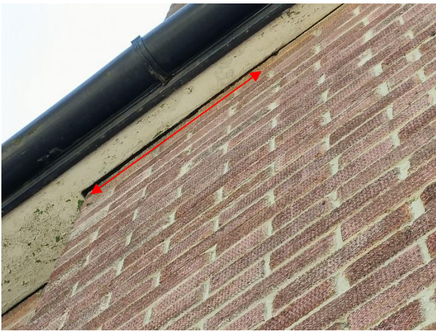
Figure 8. Example of the gaps between the soffits and the brickwork
