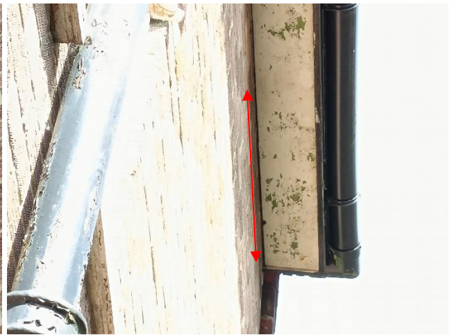
Figure 8. Example of the gaps between the soffits and the brickwork
