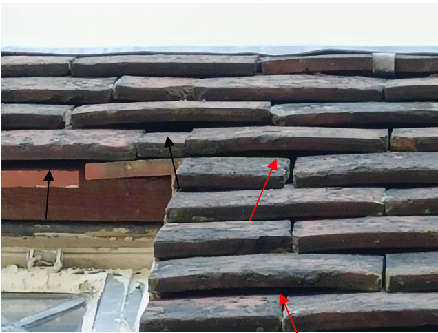
Figure 5. Example of gaps behind hanging tiles
