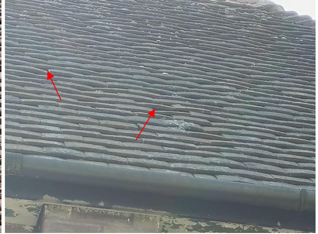
Figure 4. Example of gaps under roof tiles
