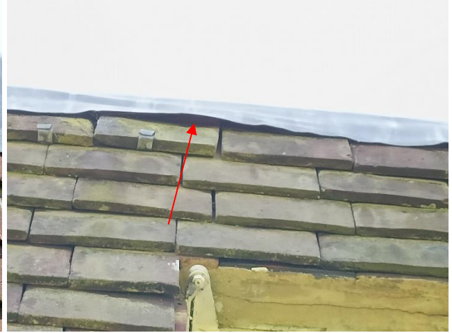
Figure 7. Example of lifted flat roof capping
