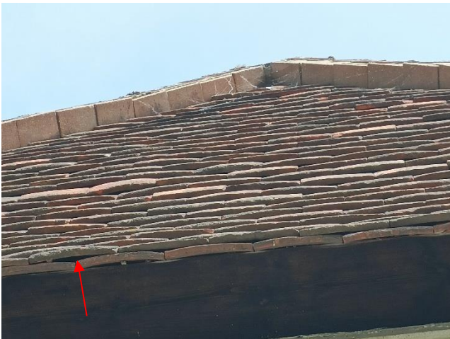
Figure 6. Example of gaps behind hanging tiles
