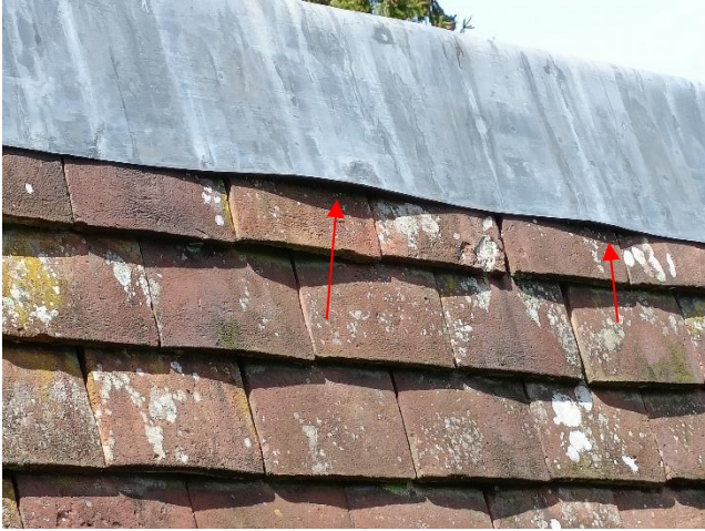
Figure 7. Example of lifted flat roof capping
